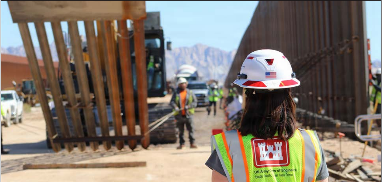
Leaders and staff from the US Army Corps of Engineers oversee BMGR-1 project construction and bollard installation, February 9, 2026, near Yuma, Arizona (US Army Corps of Engineers photo by Robert DeDeaux).
